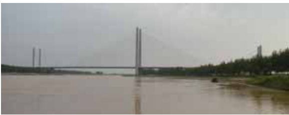
Figure 40. Photo of the Binzhou Yellow River Highway Bridge
