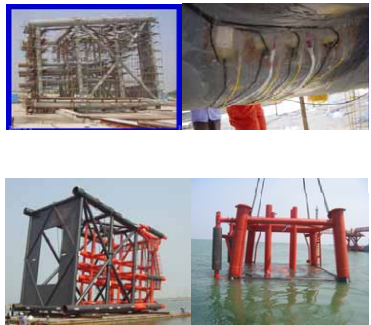
Figure39. Health monitoring system for CB32A platform
