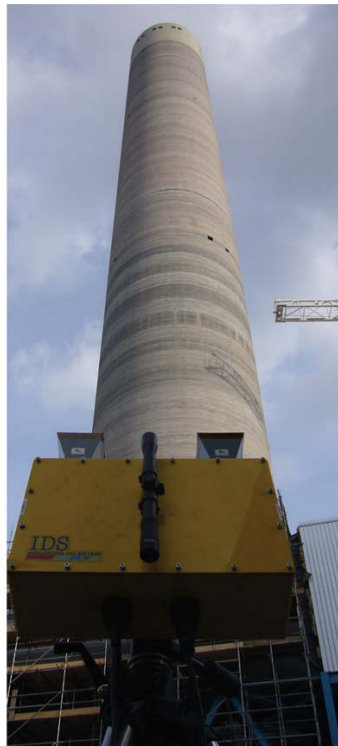
Figure 9b Radar sensor tracking new chimney
