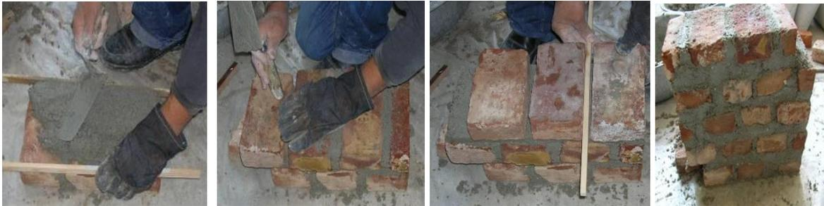
Figure 6: Construction of wall specimens
