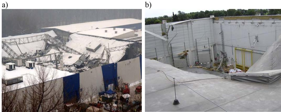
Fig. 2. Collapses due to extreme climatic loads: a - extreme snow loading, b - extreme rain water ponding of membrane covering [1]
